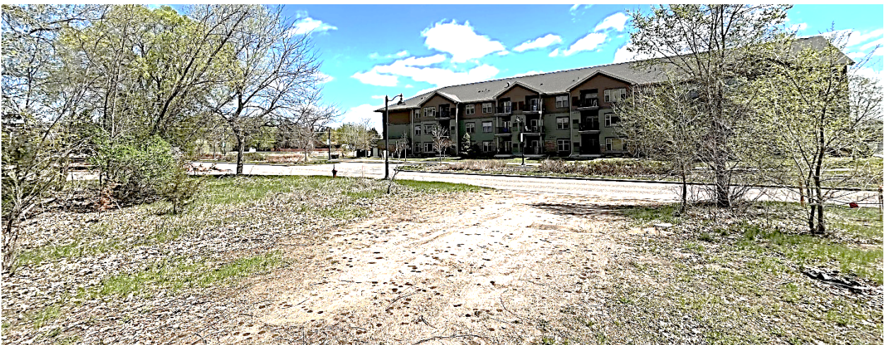
View looking east toward Balsam Apartments (Apr 30, 2026)
